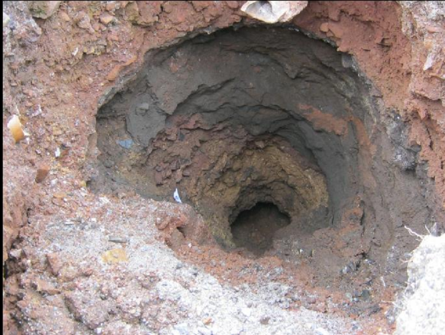
First borehole drilled into void
