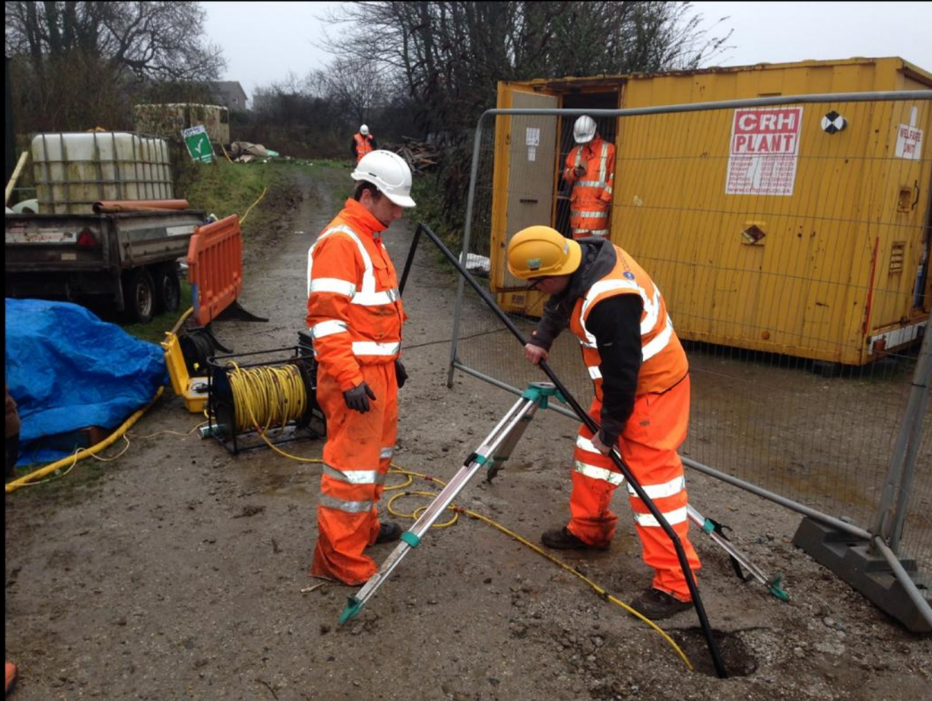
C-ALS inserted into void via borehole
