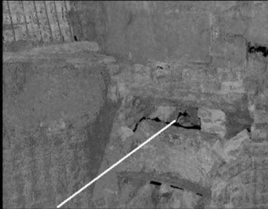
Open to adjoining chamber
